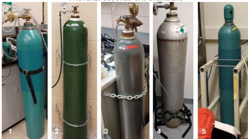
Left to right: (1) Bench-mounted single cylinder strap. (2) Two chains secured to wall. (3) Single chain at correct height secured to an immobile bench. (4) Gas cylinder stand. (5) Gas cylinder rack, valve cap in place when not in use.
