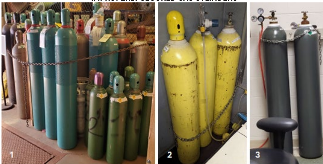
Left to right: (1) Cylinders not sorted and chained by height. Smaller cylinders not chained. Chain insufficient for the number of cylinders. (2) Chain too low on cylinders and too loose. Cylinders not nested. Cylinder on right lacking valve cap when not in use. (3) Chain too high on cylinders. Cylinder on right lacking valve cap when not in use.
